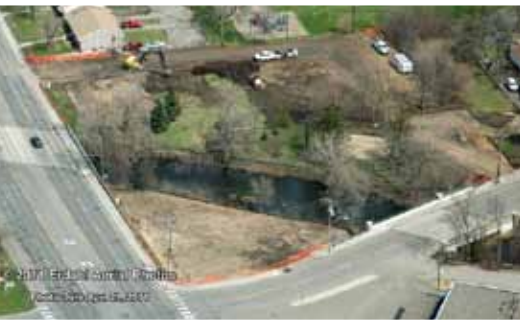
Before and after photos reveal the transformation underway at Cottageville Park.
